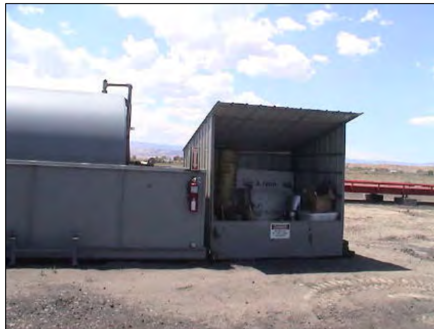
Photo 20: Non-hazardous drum storage area for petroleum products with secondary containment per SPCC Plan.
