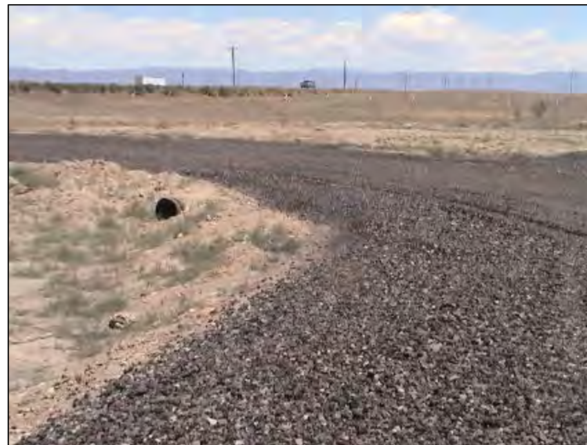
Photo 8: Internal roads consist of aggregate cover to minimize fugitive dust from mobile sources.
