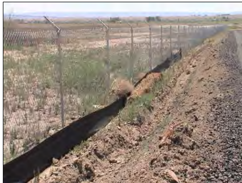
Photo 12: Silt fencing and straw bales used to complement drainage system and preclude sediment erosion off site.
