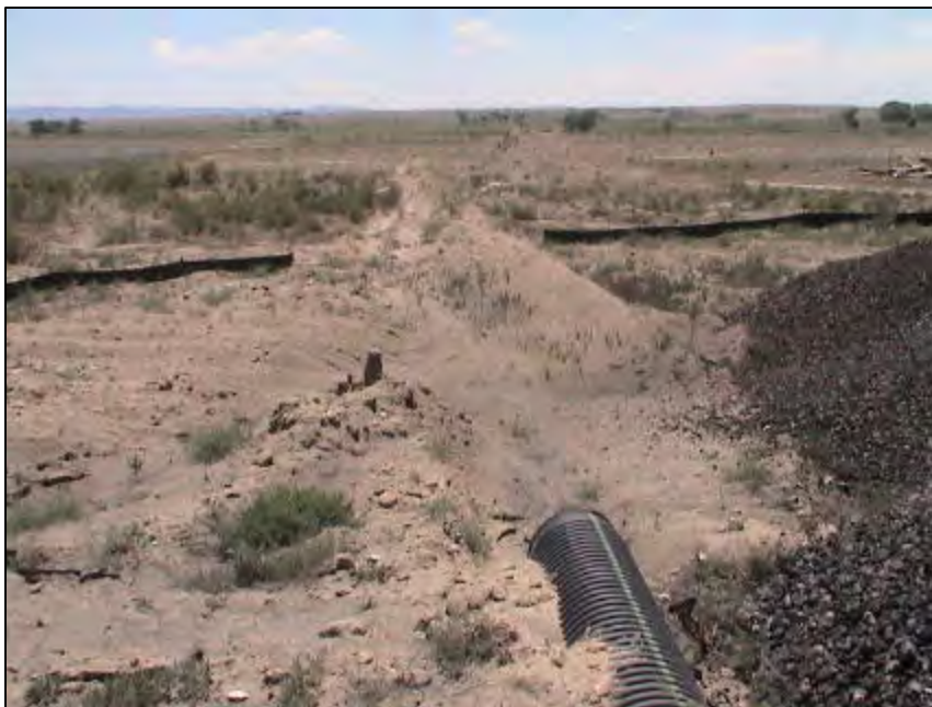
Photo 13: Drainage pipe discharges water toward storm water detention basins on south side of facility.
