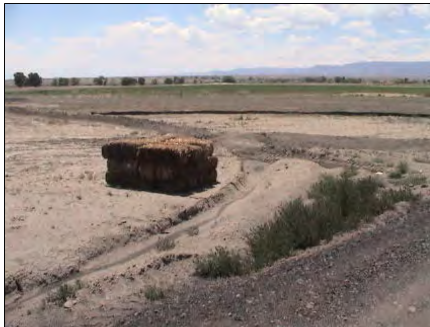
Photo 16: Drainage channel and additional straw bales (if needed) for erosion protection.
