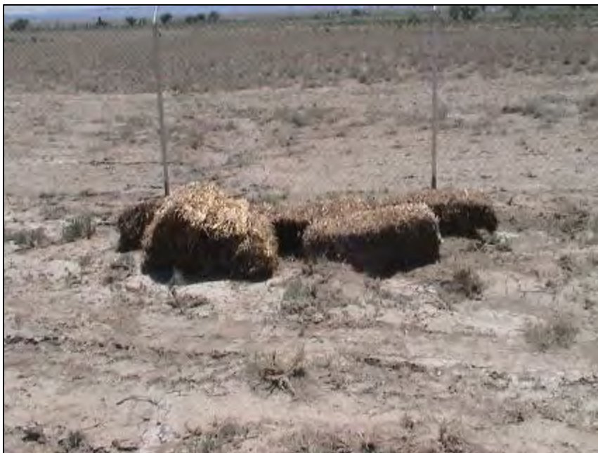
Photo 15: Straw bales used per SWPP plan for erosion protection.
