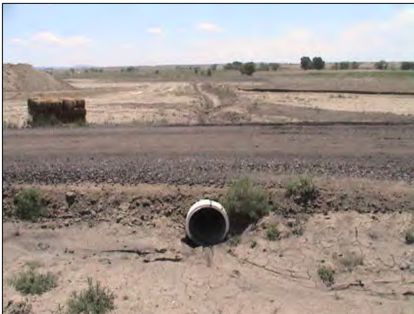
Photo 11: Storm Water managed on site using drainage channels and culvert pipes.
