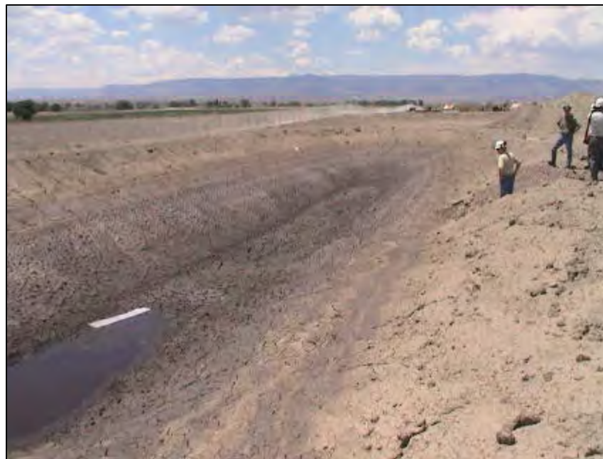
Photo 14: Storm water detention basin at southeast area of facility.
