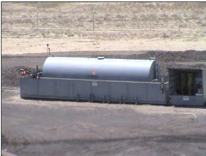
Photo 19: Diesel fuel tank with secondary containment per site SPCC Plan.
